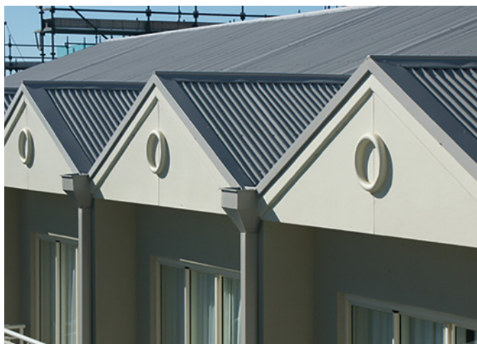
Flashings provide the essential weatherproofing at the edges, and they sharpen the image of the finished job.
